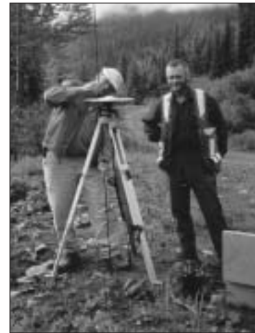
Setting up Global Positioning System (GPS) base station.
